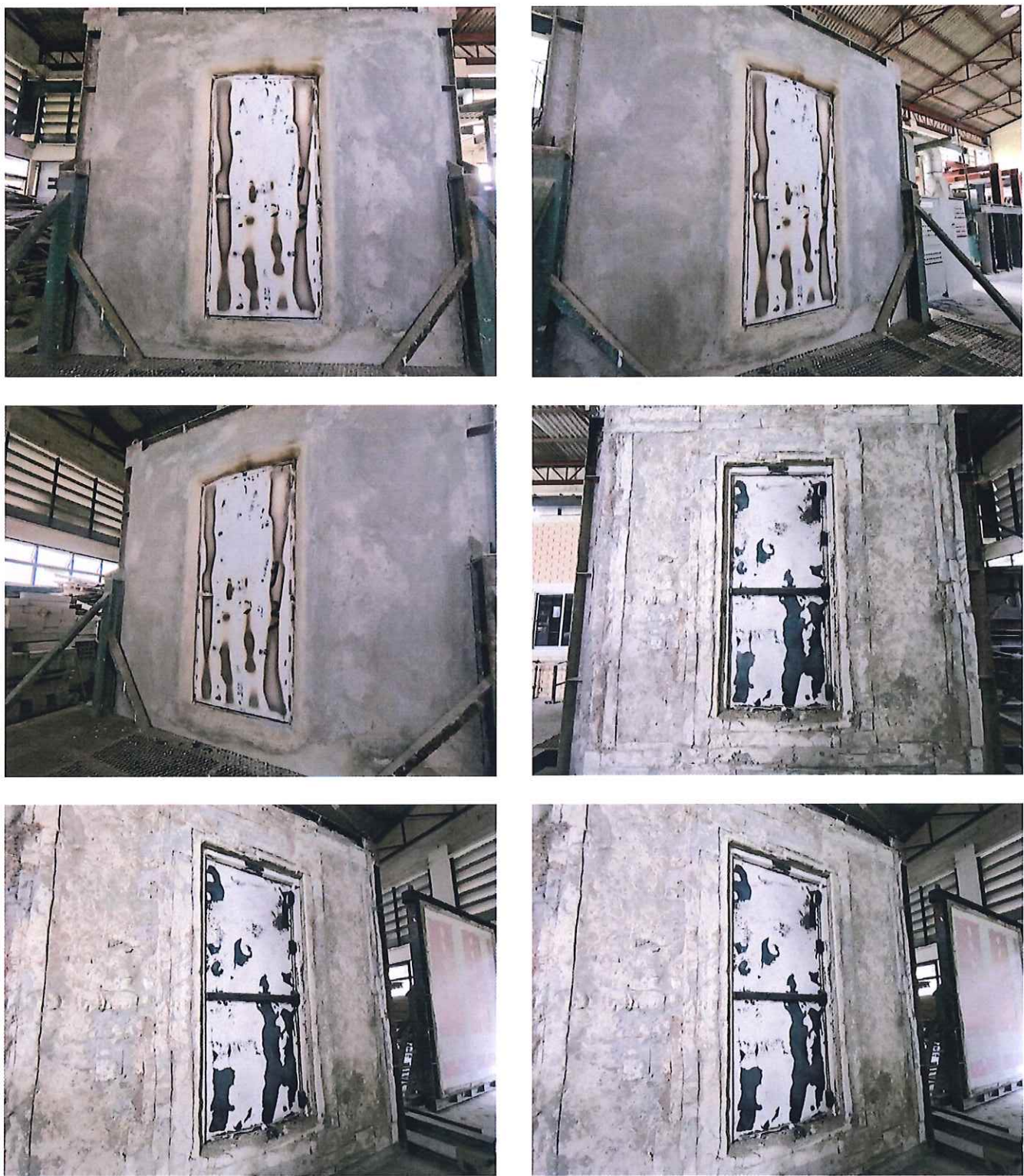
Figure D-3: The specimen after the test
